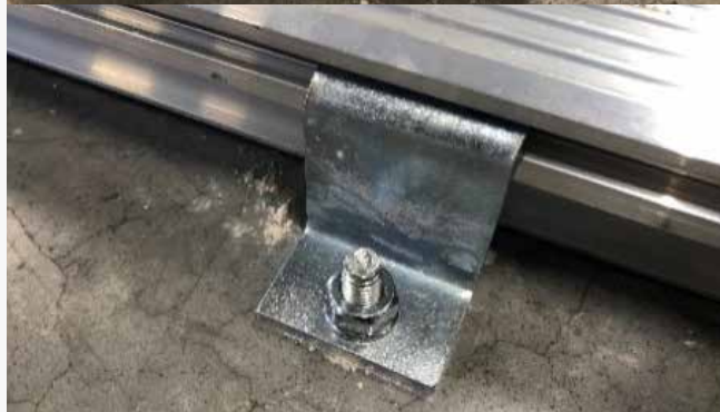
ANCHOR BOLTS AND BRACKETS
